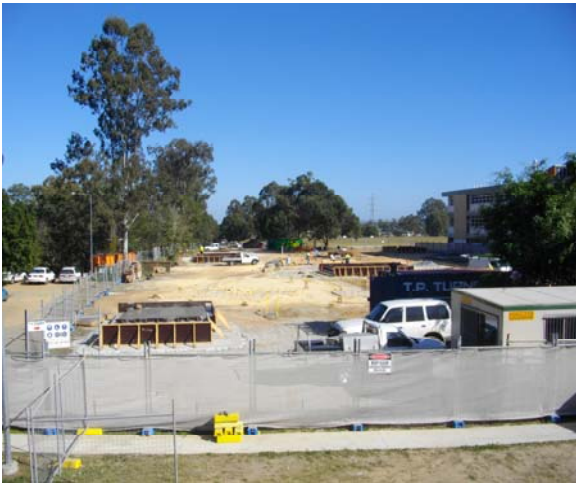
Site work - Performing Arts Centre and Leadership Centre
