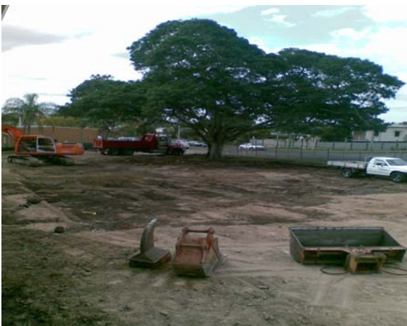
Car park redevelopment
