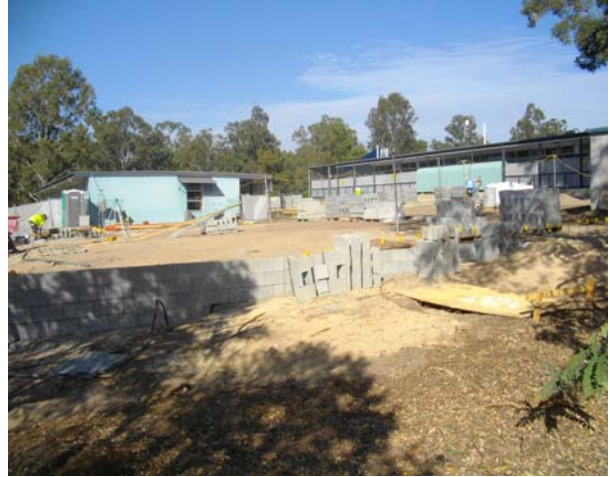
Site works for junior covered area
