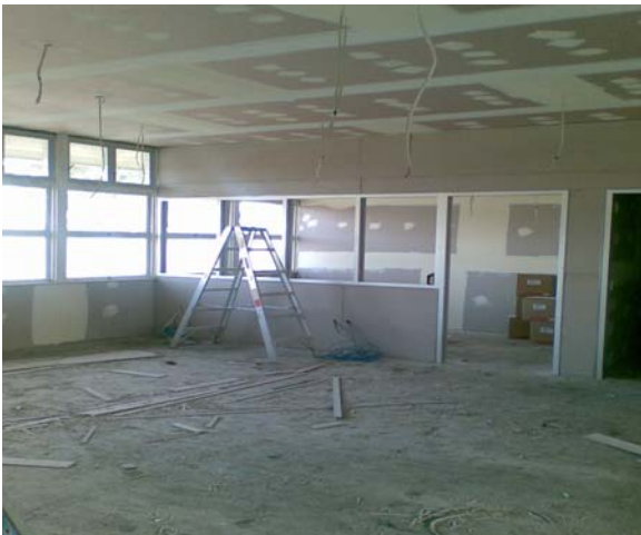
Internal refurbishment of F Block
