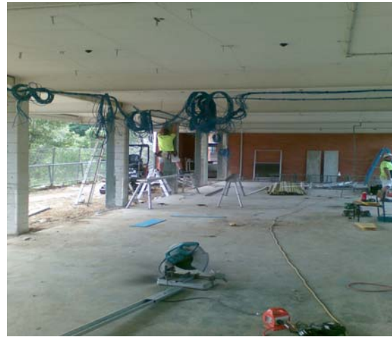
Internal refurbishment of new Special Education Unit
