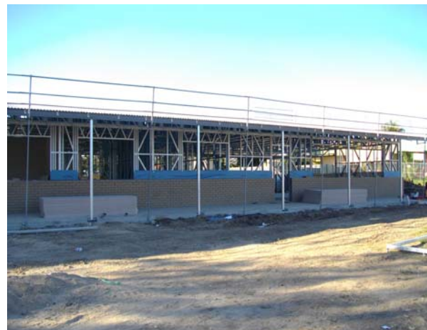
New Administration Block
