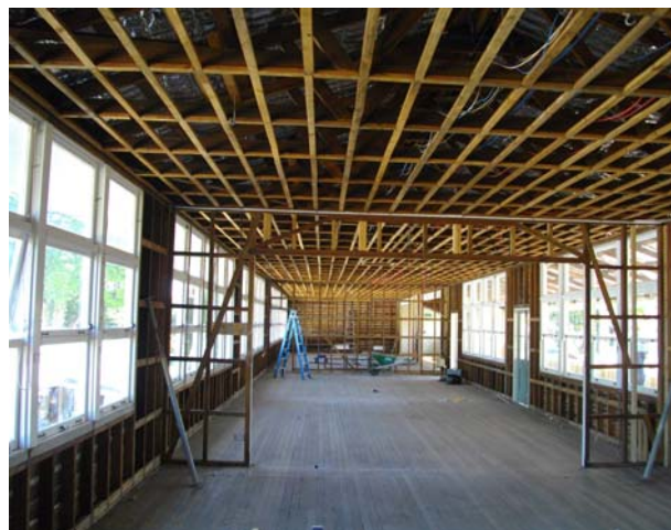
Internal refurbishment of D Block
