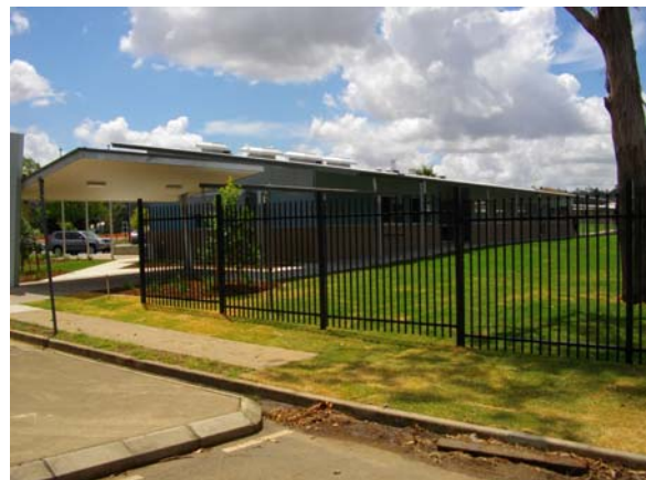
New Administration block and external fencing 266700m
