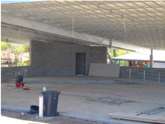
New Covered Area and stage
