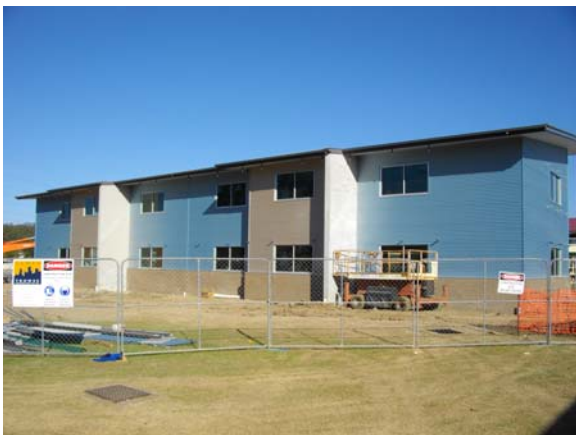
New classroom block
