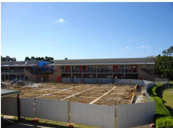
New classroom block and library foundations
