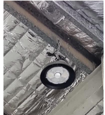
Image 1 – Example of suspended lighting fixture
